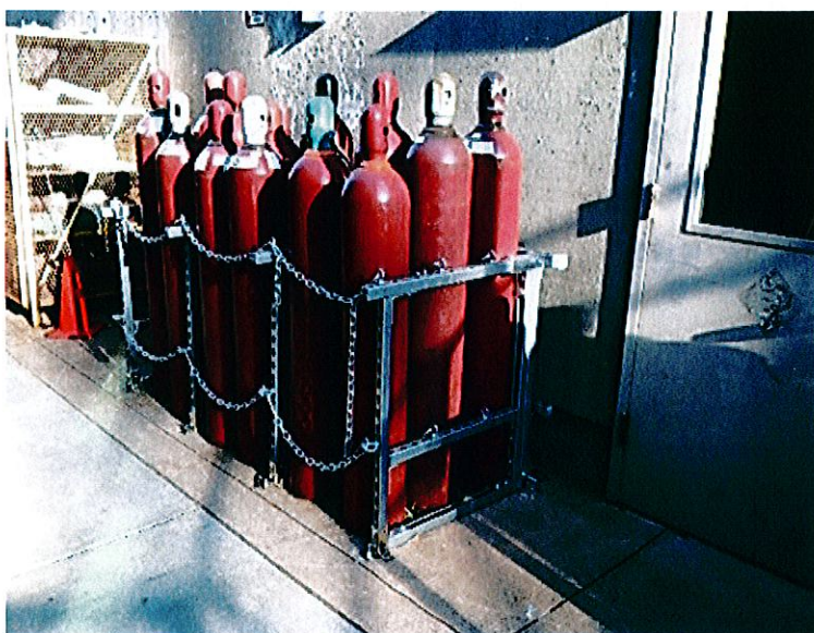
New cylinder racks flush to grade.
