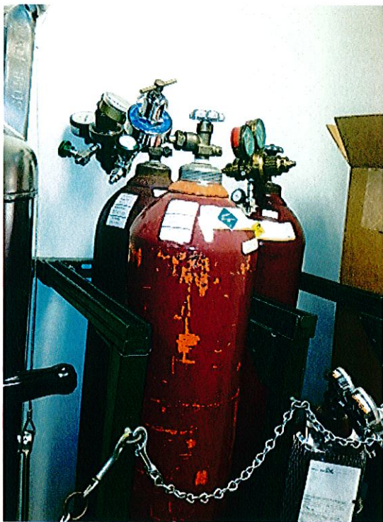
Figure 5: Cylinder storage racks originally installed with nylon straps and one set of chains. We installed second set of chains.
