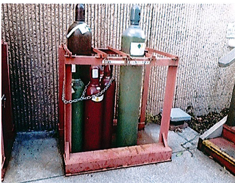
All cylinders chained to cylinder rack.
