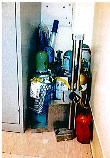
Cylinders shoved into corner and not effectively secured.
