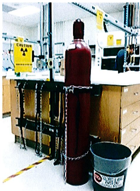
Figure 5: Cylinder storage racks originally installed with nylon straps and one set of chains. We installed second set of chains.
