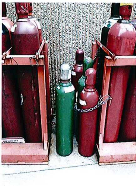
No support chains on two cylinders.
