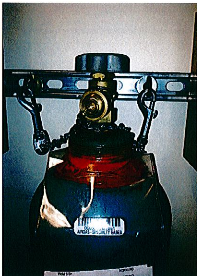
Chain support on cylinder neck, no protective valve cap.
